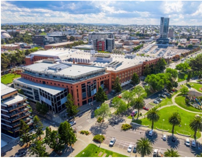
Deakin University Waterfront Campus, Geelong, Victoria (Credit: Deakin University, 2026).
